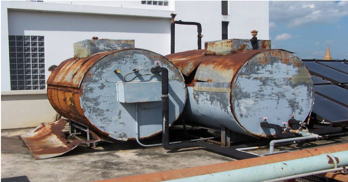
Figure 3.1 Picture of a neglected solar system In Thailand
